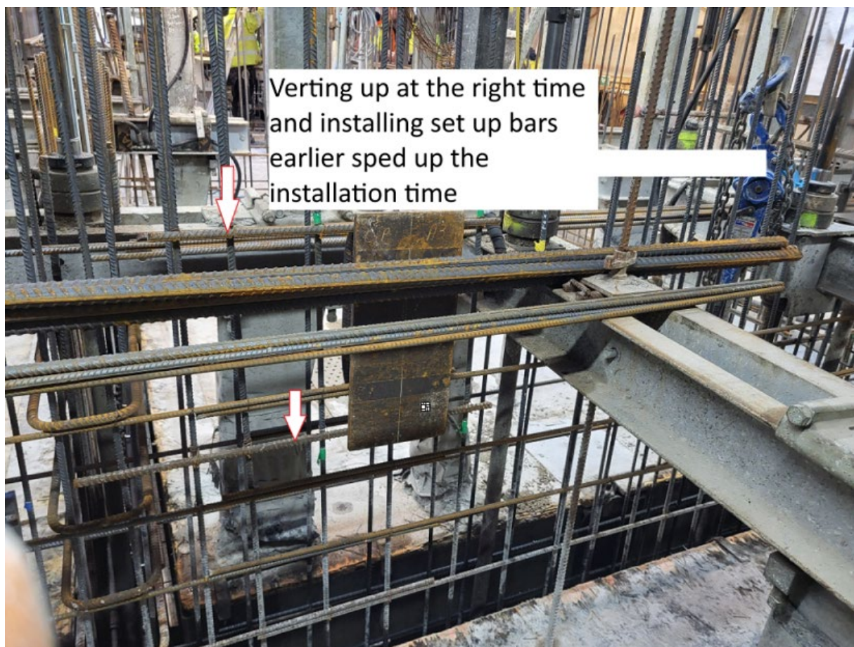
Figure 5 Embedment plates technical solution
