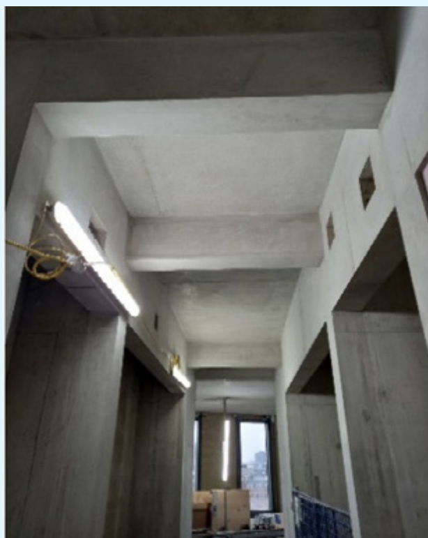
FIGURE 1 – Lobby slab/beam with Elder Yard core
