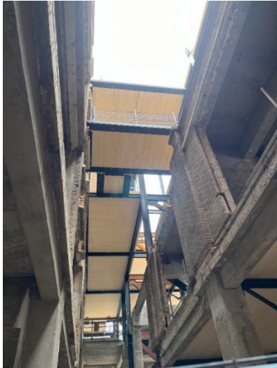
Figure 16 Image showing typical connections between old and new structure
